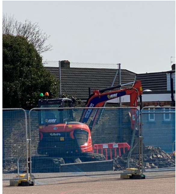
JCB digging the foundations
